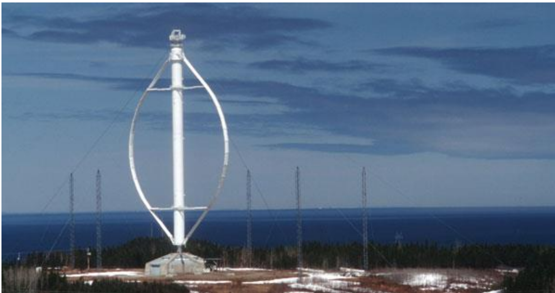
Figure 2:3: Darrieus Turbines [6]
